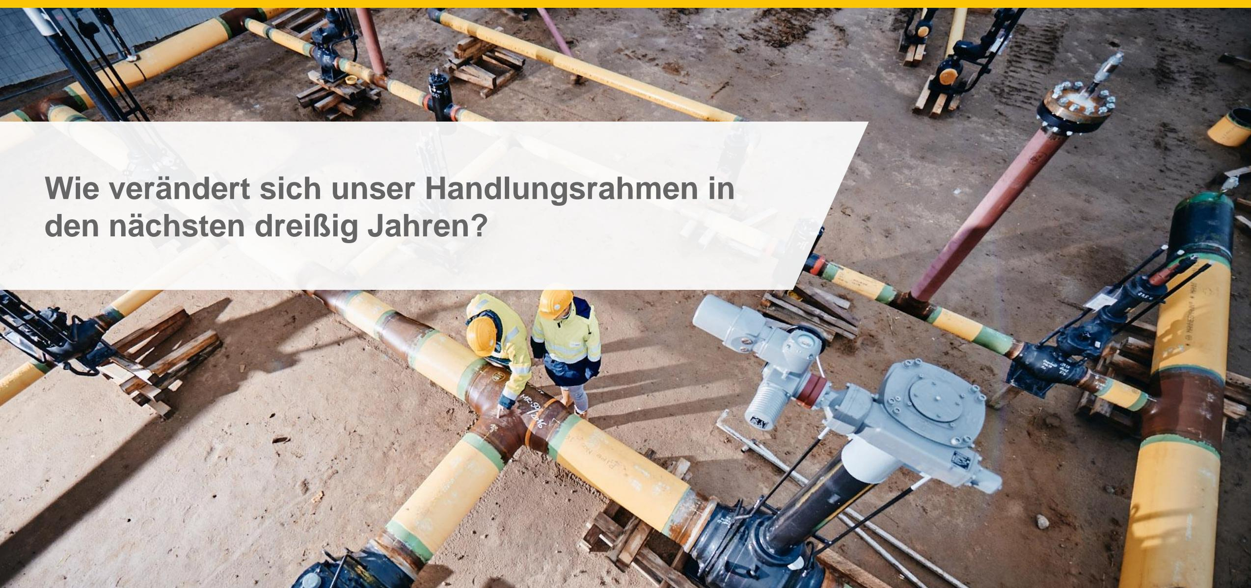
An aerial photograph of an industrial gas pipeline construction site. The ground is dirt. Several large pipes are laid out, some painted yellow with green and brown sections. Two workers in high-visibility yellow jackets and hard hats are standing near a pipe. In the foreground, there are large grey valve actuators. The scene is brightly lit, casting shadows.
